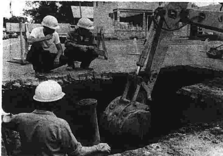
Water department crew hunting for a break in a water main.
